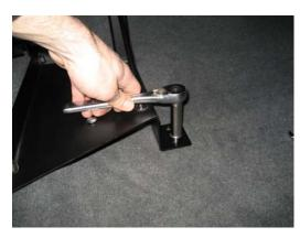
Attach bracket to floor using ¼" x 1" hex head lag bolts
